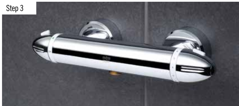
Step 3 Install the concealing plates so they are flush to the wall. Offer the bar valve up and secure.
